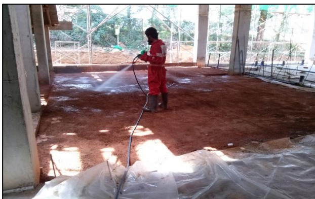
Figure 2.1: Anti termite treatment
